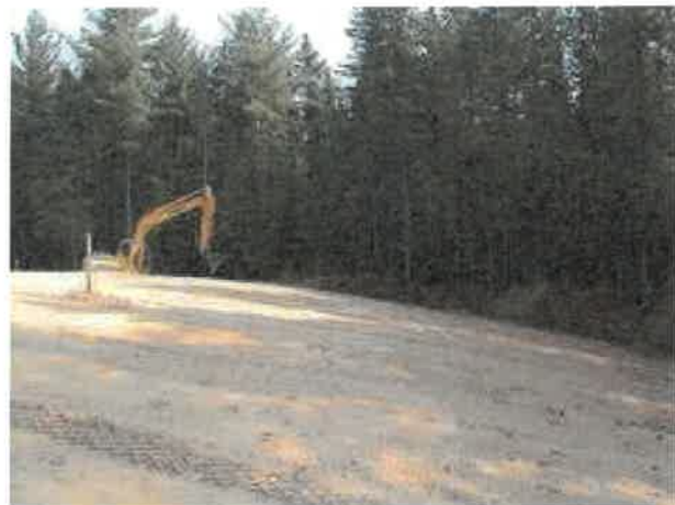
A construction project involving soil disturbance
